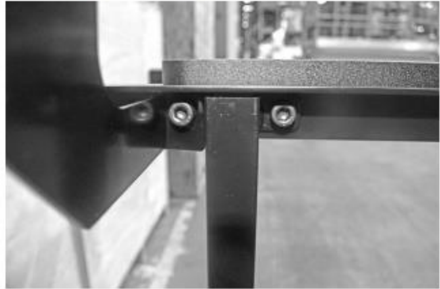
Hose support and Leg properly Installed:
